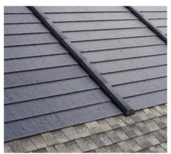
Timberline Solar® ES 2 installs alongside any Timberline® asphalt shingle, using the same crew, tools, and expertise.
